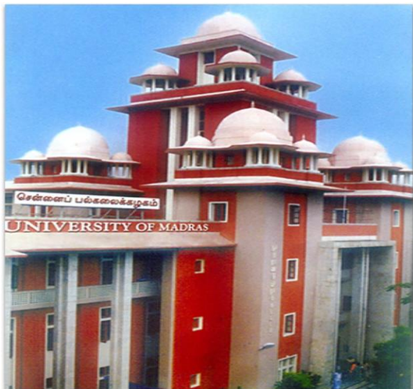
Centenary Building Chepauk Campus
